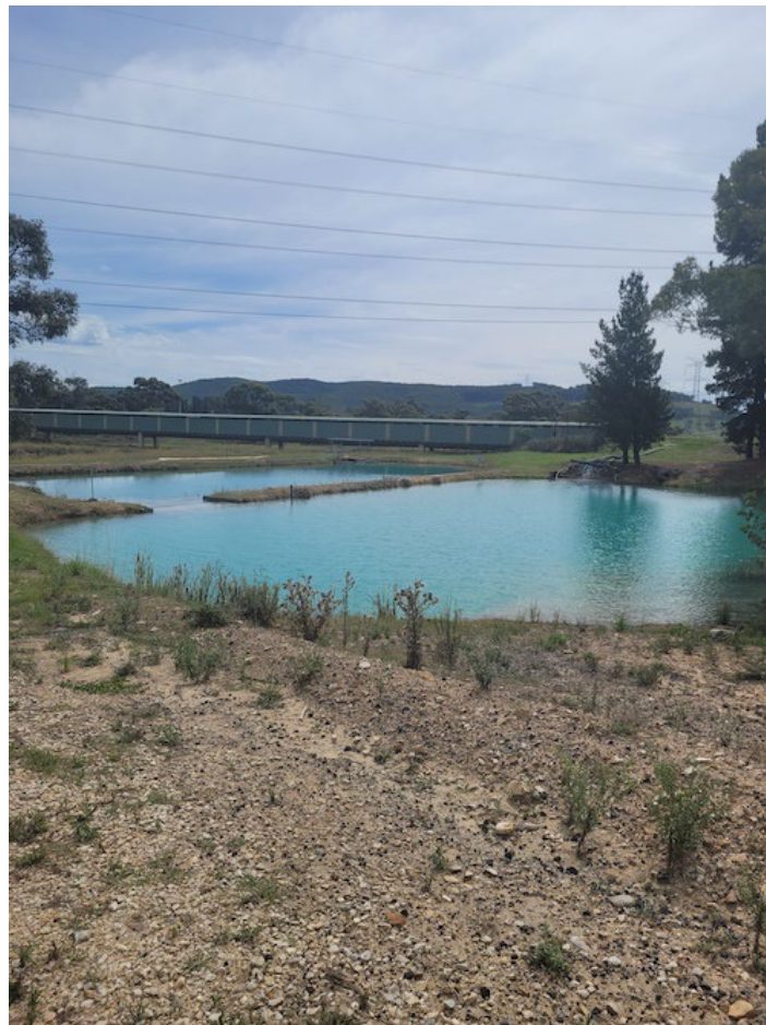
Clean Water Discharge Final Settling Ponds
