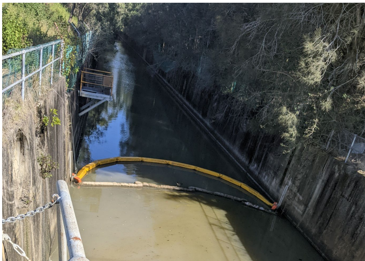
Sediment and Contamination Booms Within Hammond Canal
