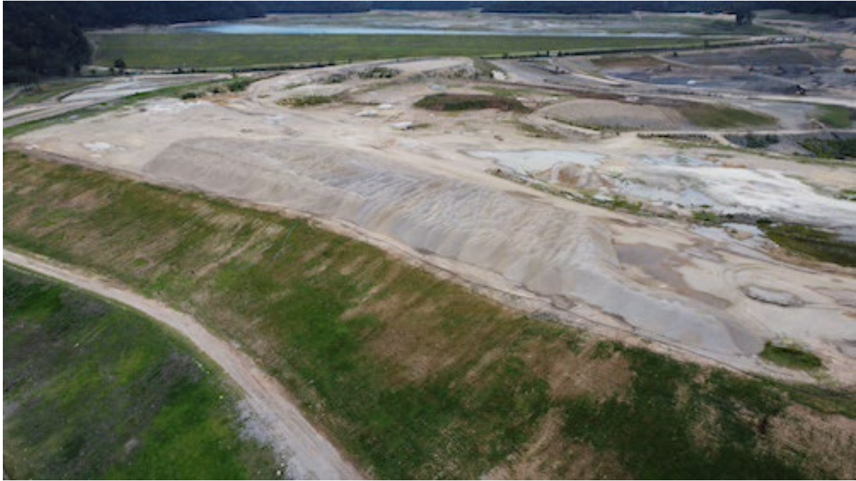
Hydromulching Sprouting on the Wall of KVAR
