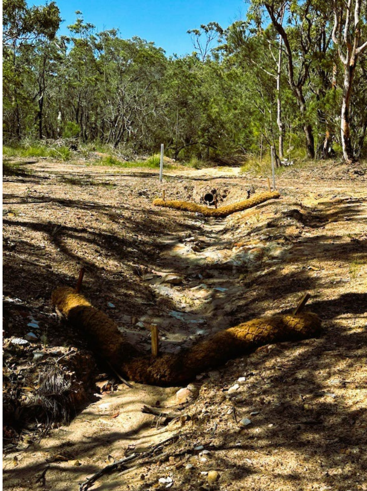
Sediment Controls Within Drainage Channels
