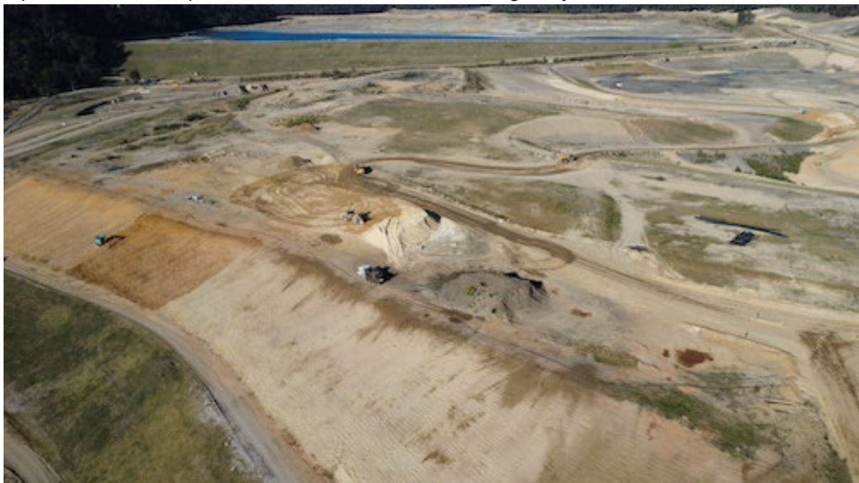
Hydromulching and Stockpiles on KVAR
