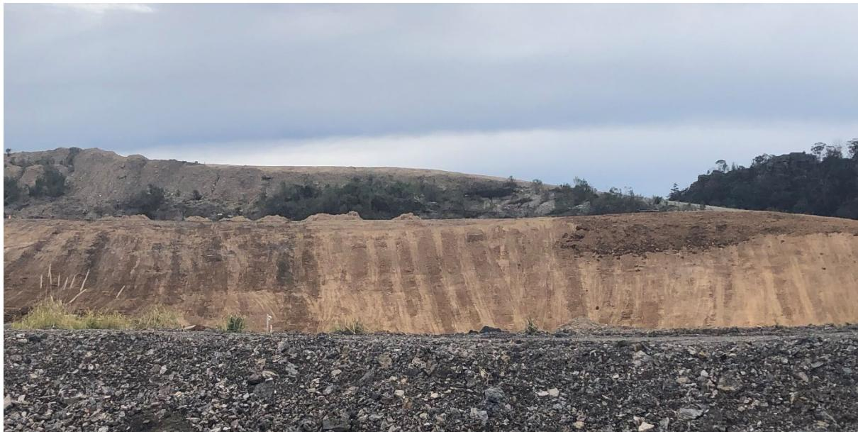
**Photograph 8.3**      **Regrading of KVAR berms**
