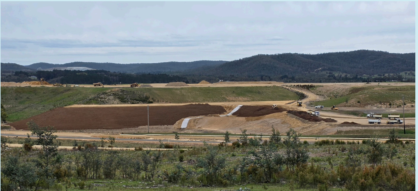
Figure 3: Slope stability works with erosion and sediment controls
