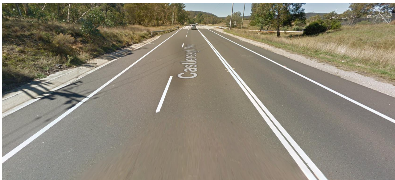
Photograph 2.1 Castlereagh Highway (looking eastbound near site entrance)
