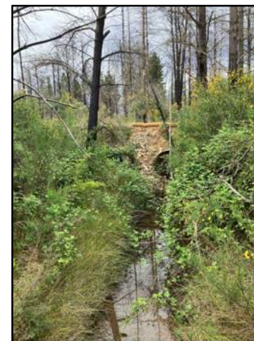
CULVERT 5 (UPSTREAM END) (LOOKING NORTH)
