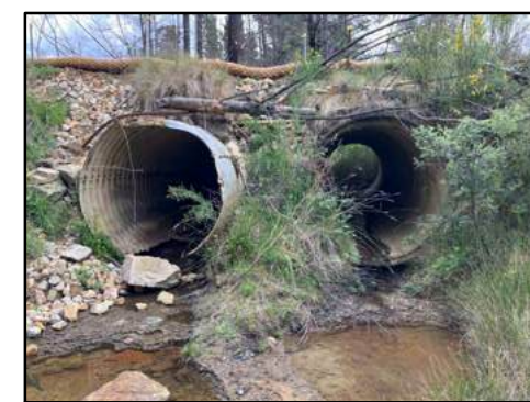
CULVERT 5 (DOWNSTREAM END) (LOOKING SOUTH)
