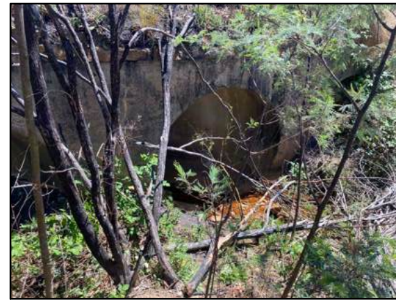
CULVERT 1 (UPSTREAM END) (LOOKING WEST)
