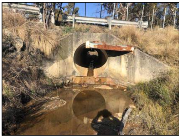
CULVERT 2 (DOWNSTREAM END) (LOOKING EAST)
