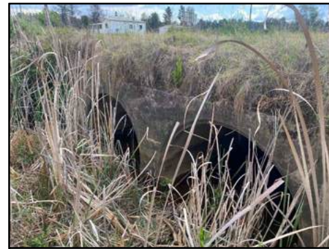
CULVERT 3 (UPSTREAM END) (LOOKING WEST)
