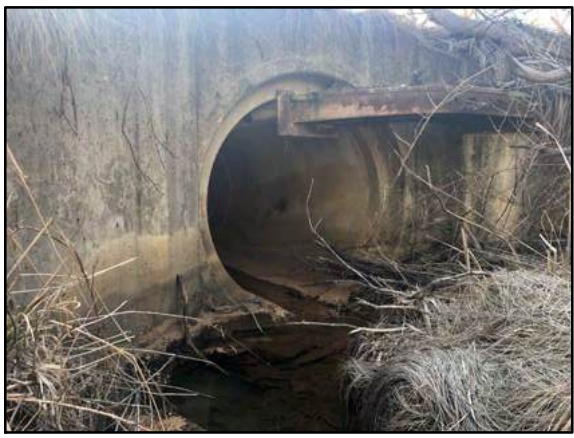
CULVERT 2 (UPSTREAM END) (LOOKING WEST)
