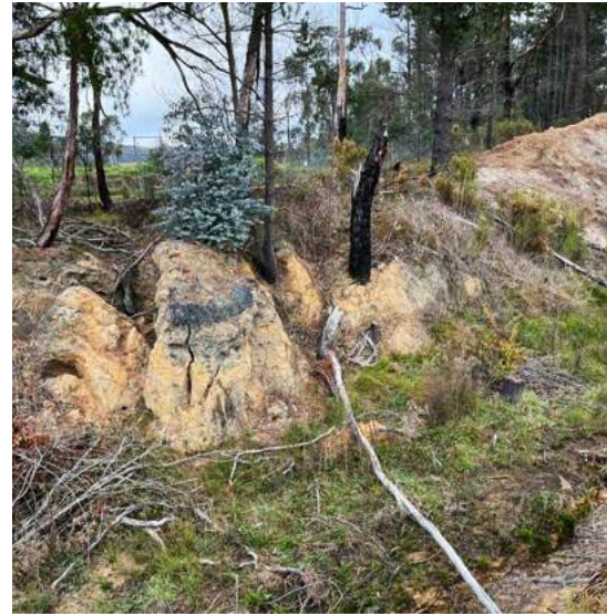
Eastern channel bank, adjacent to Lidsdale Cut – downstream of Stage 1
