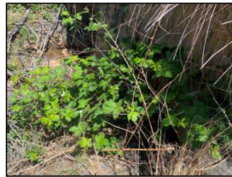
CULVERT 3 (DOWNSTREAM END) (LOOKING EAST)
